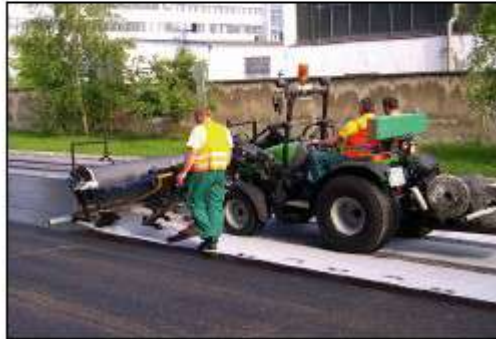
Laying of Geogrids are in progress
