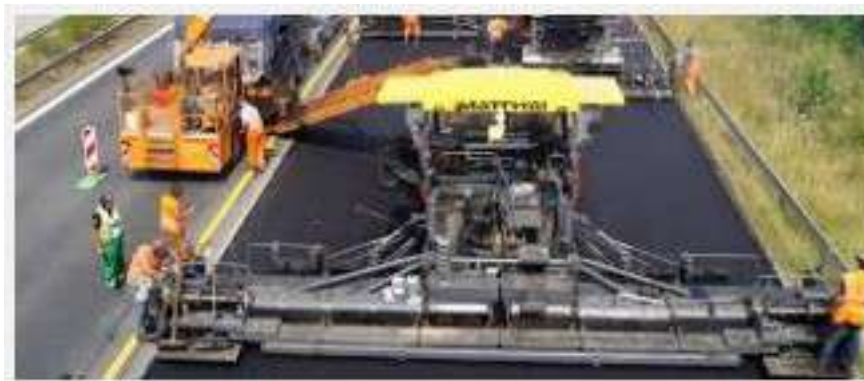
Pavement construction for Road Widening
