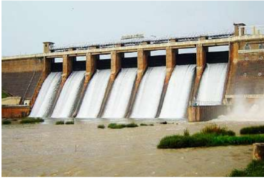
Discharge from the Dam
