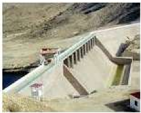
Concrete Gravity Dam
