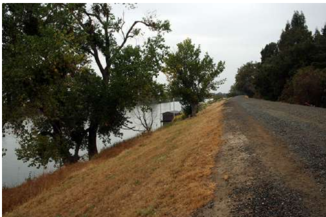
Earth Dam / Dyke
